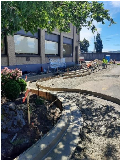
1 Before curb, sidewalk, & ADA ramp
