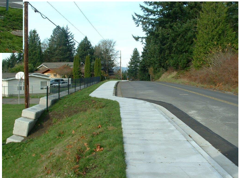
Military Road Sidewalk Improvements completed in 2012
