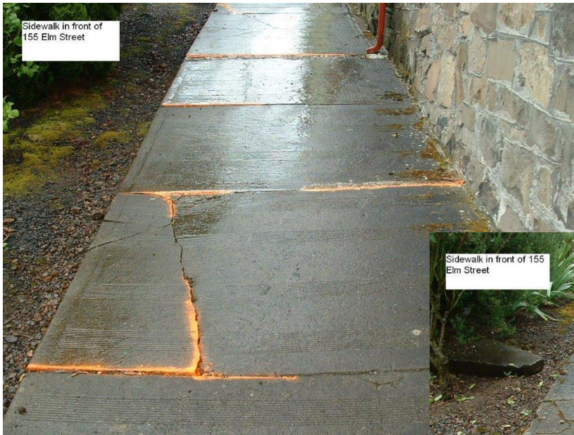
Elm Street Sidewalk Improvement Project - Slated to be completed in 2013 -2014
