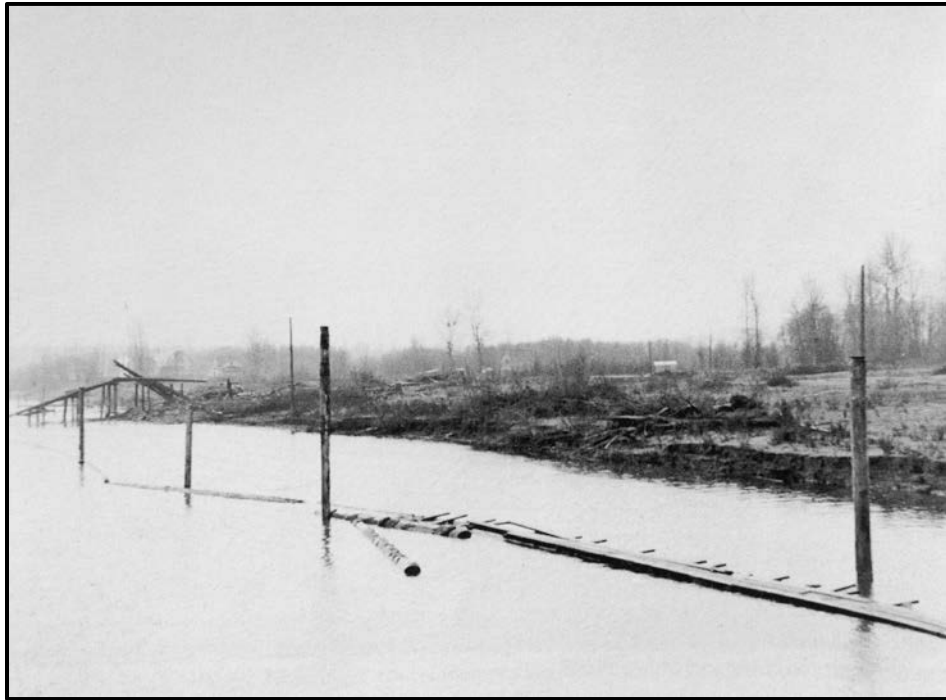
Figure 16. North-facing photo of timber piles for mooring log rafts off the Kalama shoreline, early 1900s (Thomas 2016).
