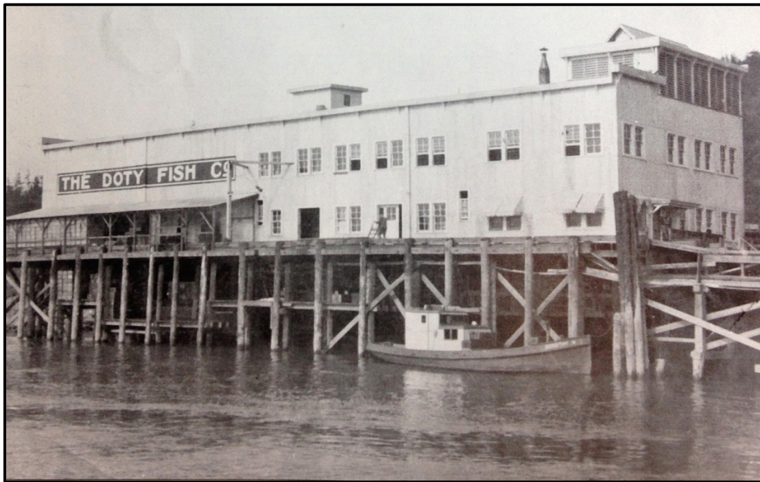
Figure 9. Northeast-facing photograph of the rebuilt Doty Fish Company building (undated but post-1924) (Thomas 2016:48).
