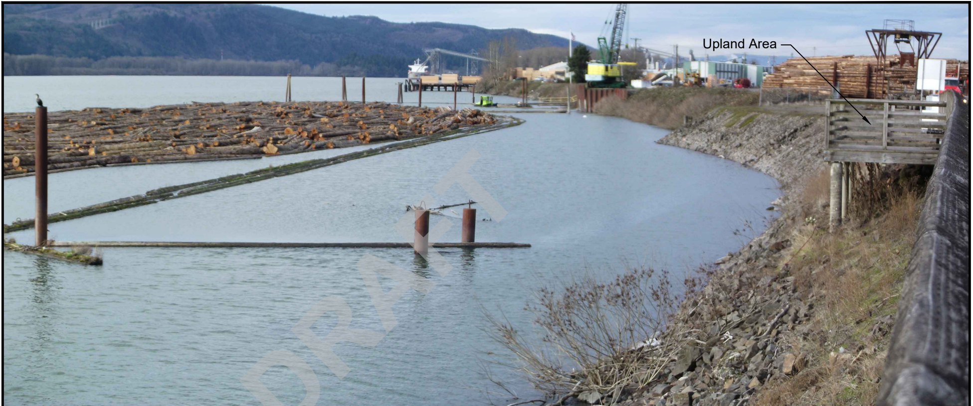
Looking at the existing log storage area and shoreline conditions. The proposed upland area is on the right side of the photograph. Pile caps will be installed on all new and relocated piling to prevent bird perching.
