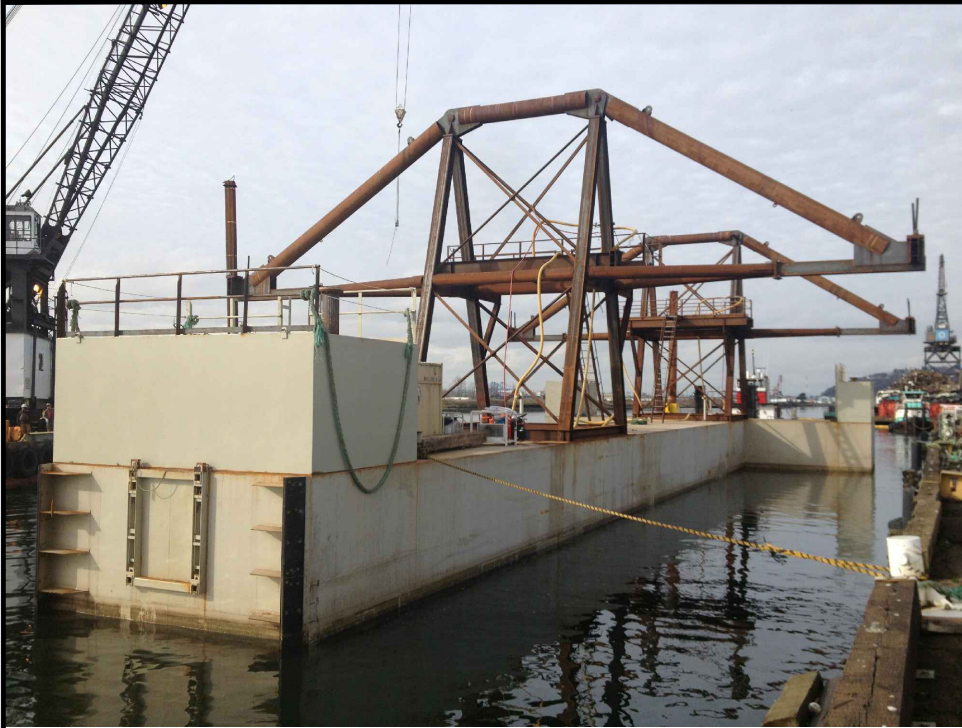
Photograph of T-barge. Framework above the deck has been removed.
