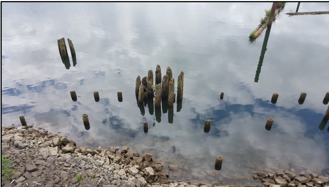
Figure 7. Southwest-facing view of the southernmost piles proposed for removal.
