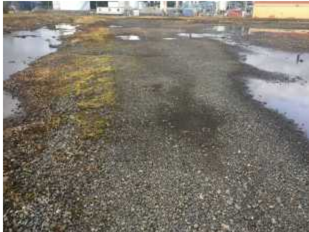
Picture of existing gravel fill material covering storm pond area.
