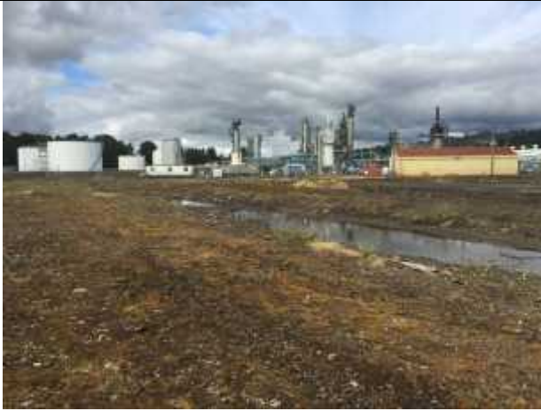
Storm pond area looking northeast.
