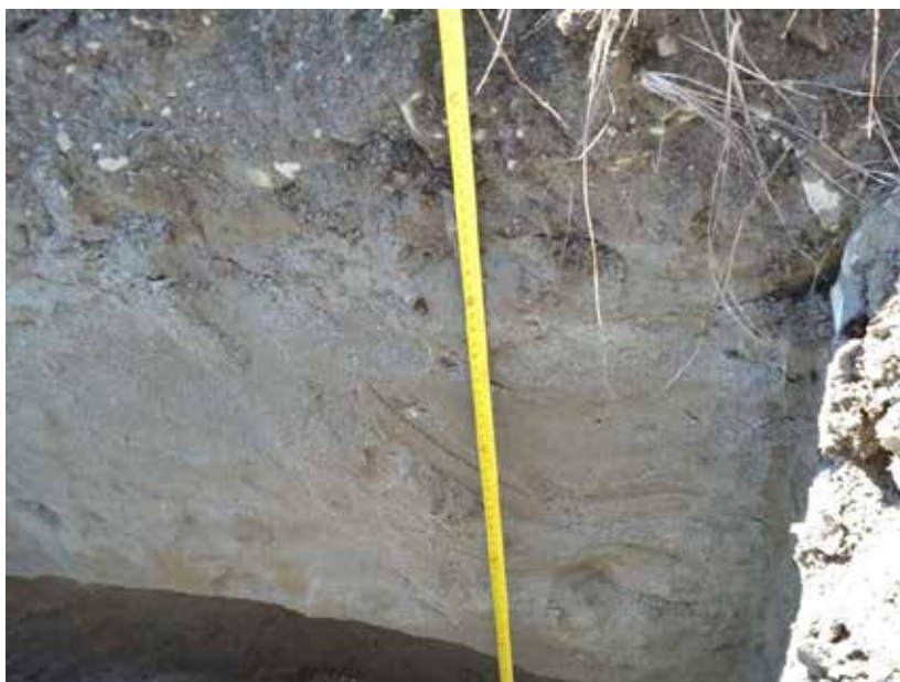
Photo 5. Profile of test pit TP-3 to a depth of 3.2 m (10.5 ft). The view is towards the south.
