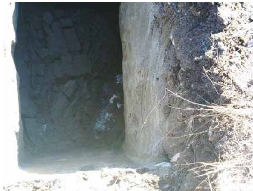
Photo 8. Overview of test pit TP-2 with water at the bottom of the test pit. The view is down and towards the northeast.
