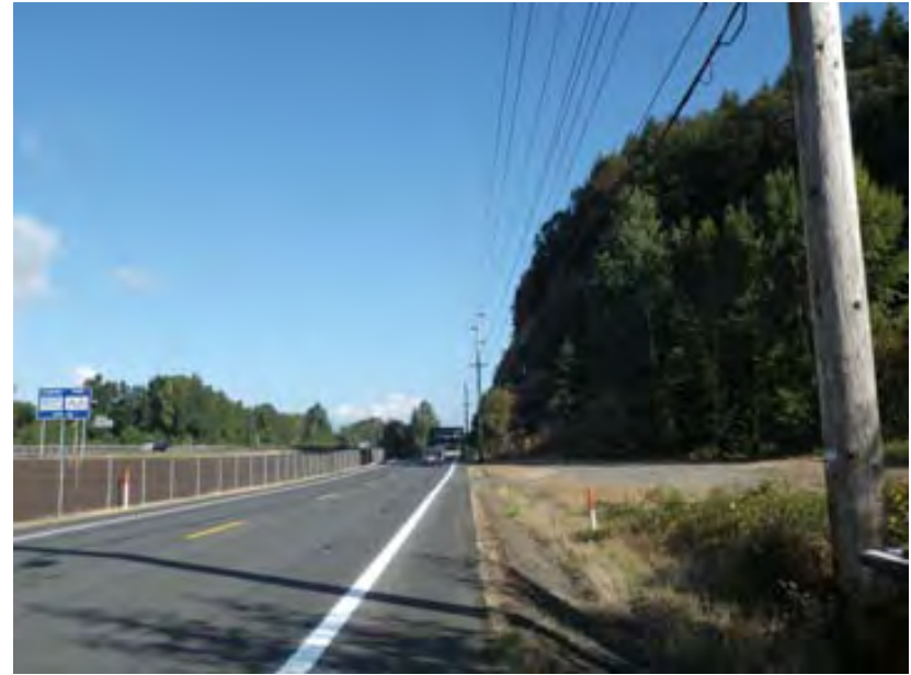
Photo 6. The project area from its southernmost point. Note the fence and trenched utilities on both sides of Meeker Drive. The view is towards the north.
